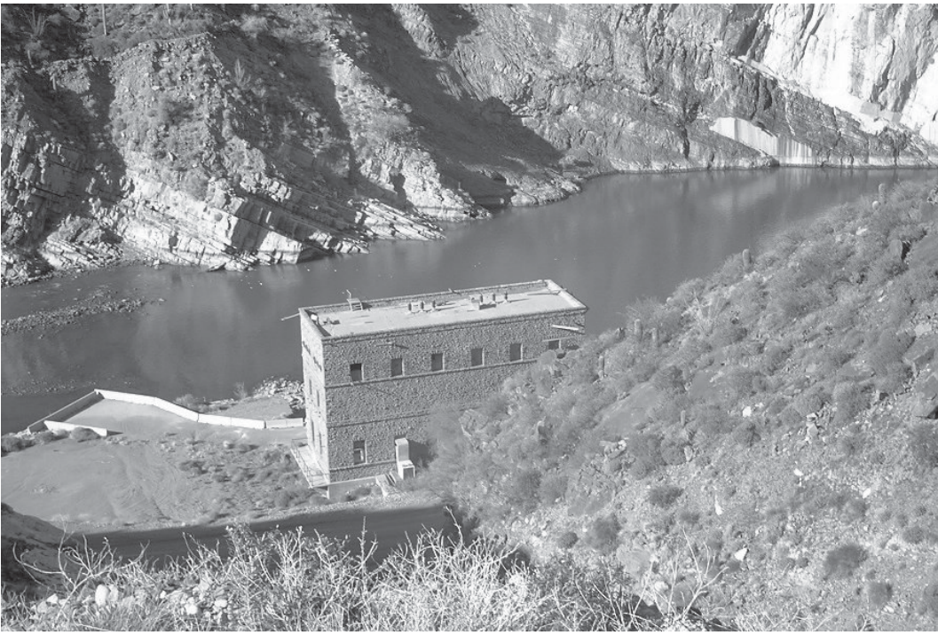
Old powerhouse at Roosevelt Dam
